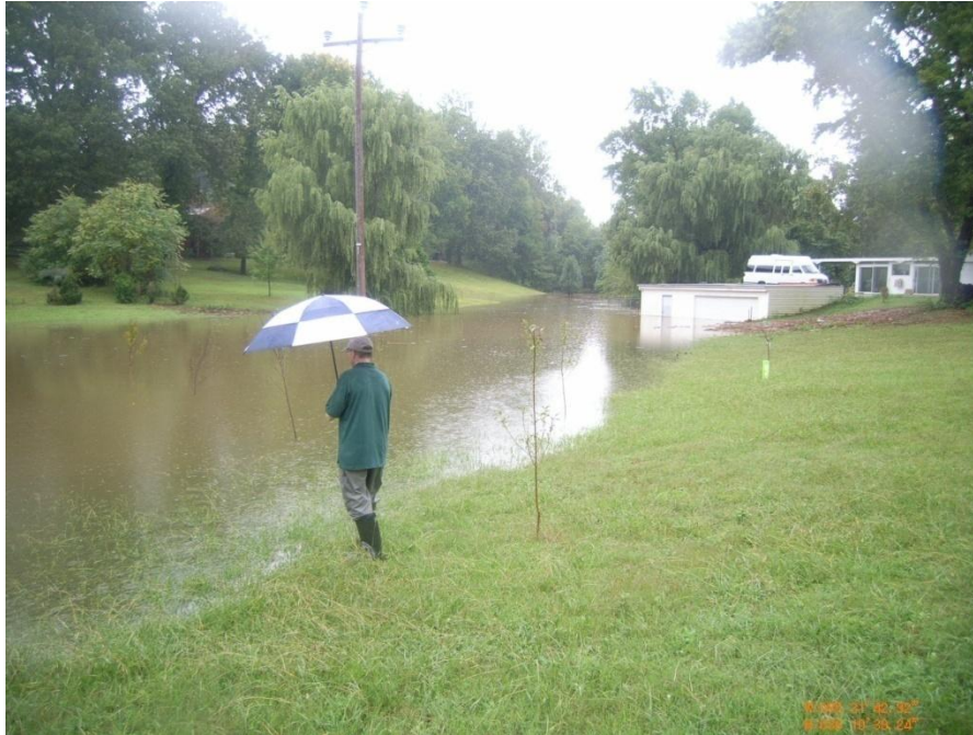
Figure 11. Flooding near the intersection of West 9 th St and Hawthorne during 9-16-09 storm.
